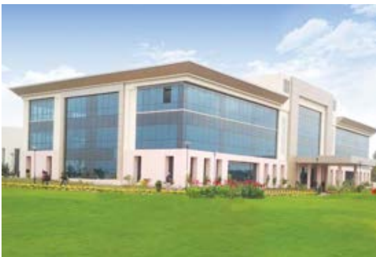
Switchgear Factory, Vadodara
