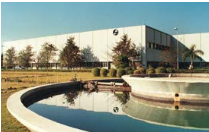
Switchgear Factory, Ahmednagar
