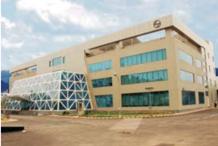
Switchgear Factory, Navi Mumbai
