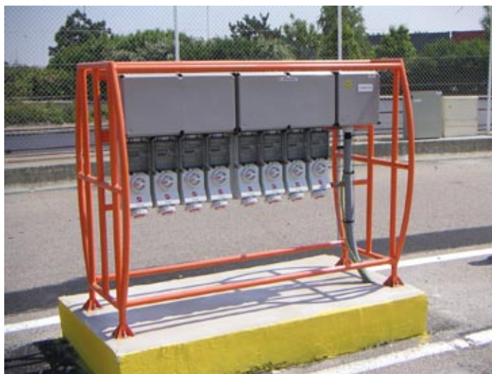
Container Terminal, Le Havre – France
